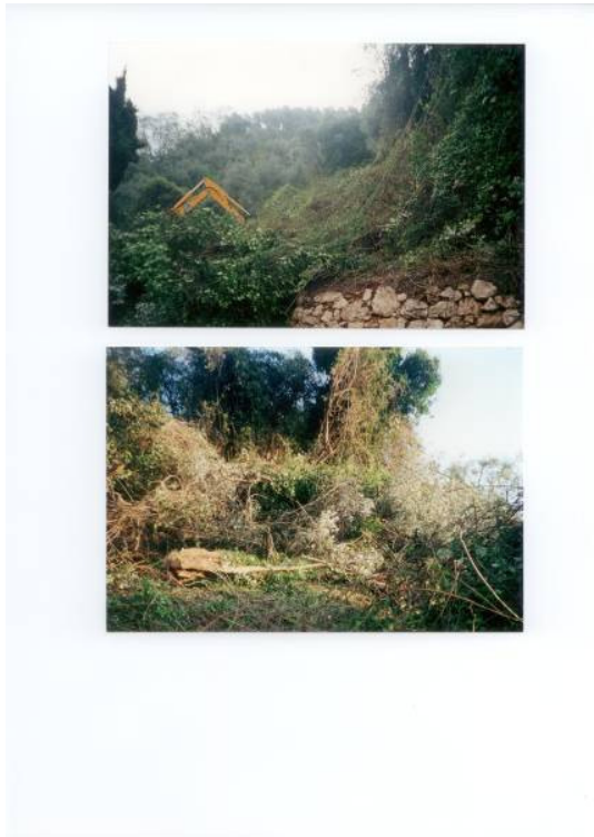
Fig. 7 State of the olive grove when the works began
